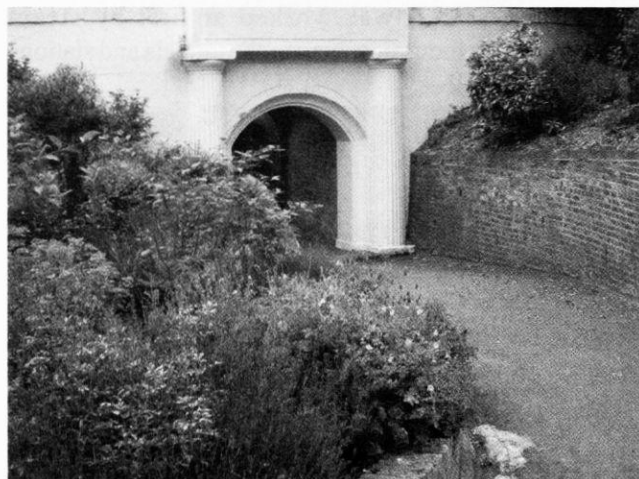
North Portal – Photo by Drew Bennelick
